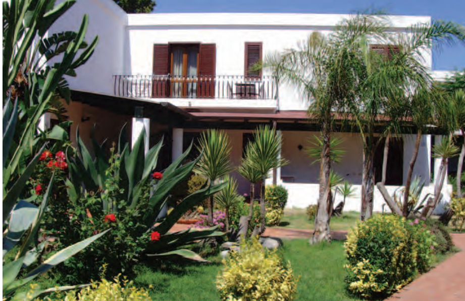
Residence la Giara
